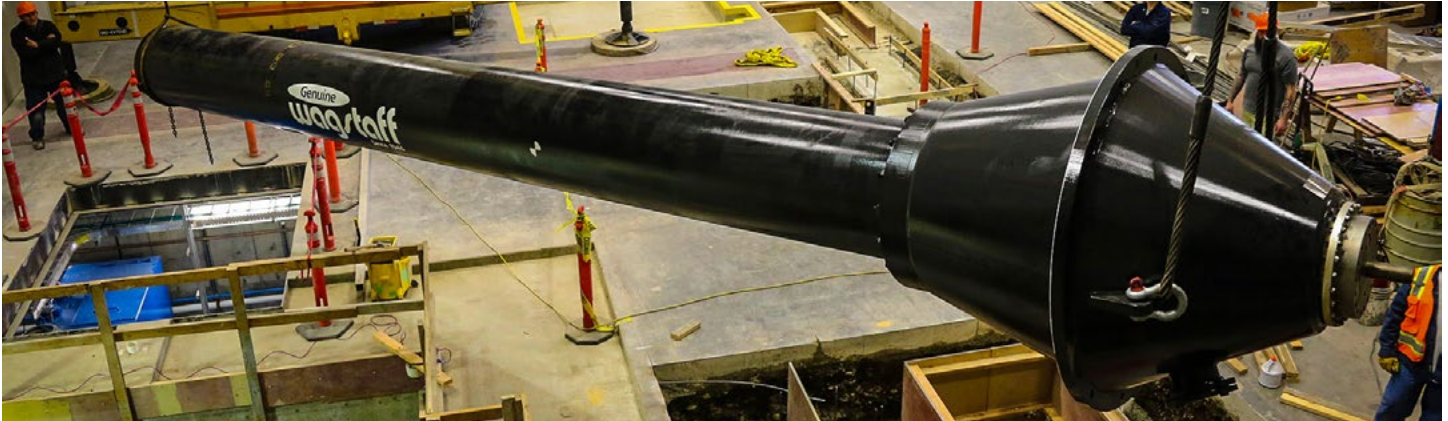
A Wagstaff casting cylinder being installed.
