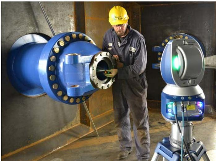
“We’ve just started designing a 25-megawatt Pelton turbine in British Columbia,” says Graves. “Alignment of a system of this size is traditionally done with jigs, lasers, and levels. A laser tracker will help us verify our manufacture and install the equipment with precision, much quicker than with these traditional methods—especially with the physical scale we’re working with.”
