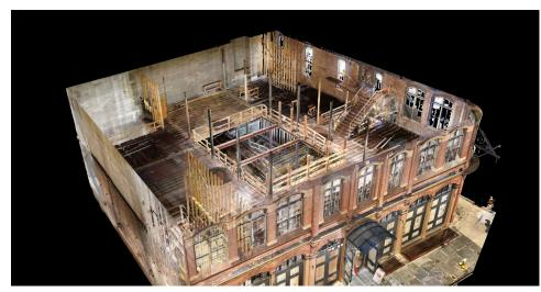
FARO® Laser Scanners and As-Built™ software were instrumental in modeling the Wagener Building.
