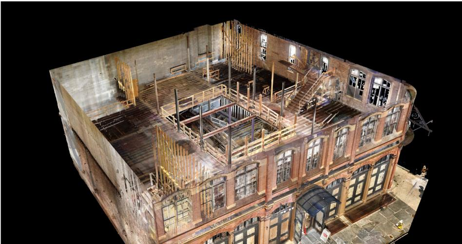
FARO® Laser Scanners and As-Built™ software were instrumental in modeling the Wagener Building.
