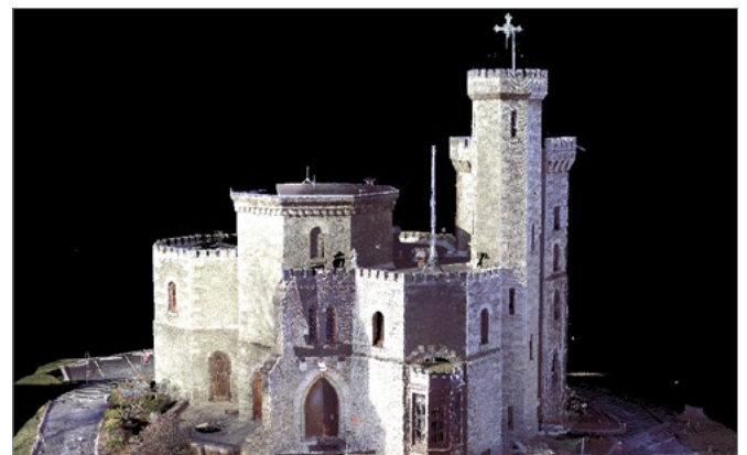
Figure 2. The completed exterior scan project via SCENE Software.
