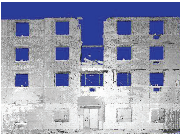
Figure 7. Scan data of the collapsed building under construction.
